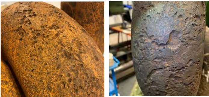
Figure 1: Mooring chains surface condition due to corrosion
