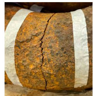
Figure 4: Main fracture in lower crown of LINK 1
