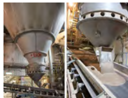
Figure 2: Hopper lays out raw ingredients
