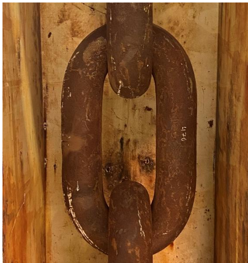
Figure 1: Mooring chain sample showing corrosion
